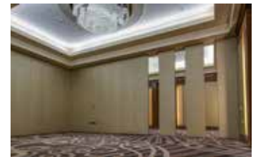
Panels nest deeply and seal tightly to create an acoustic barrier with a rating of 56 STC - the highest in the industry.
